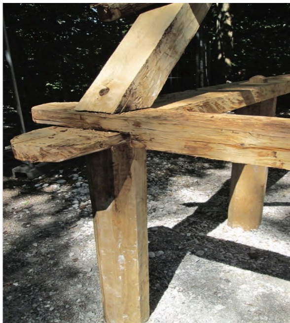
Details of the corner of the building showing dowels.
