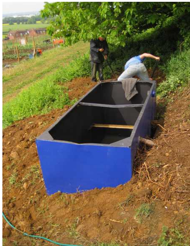
First water tank now installed and levelled
