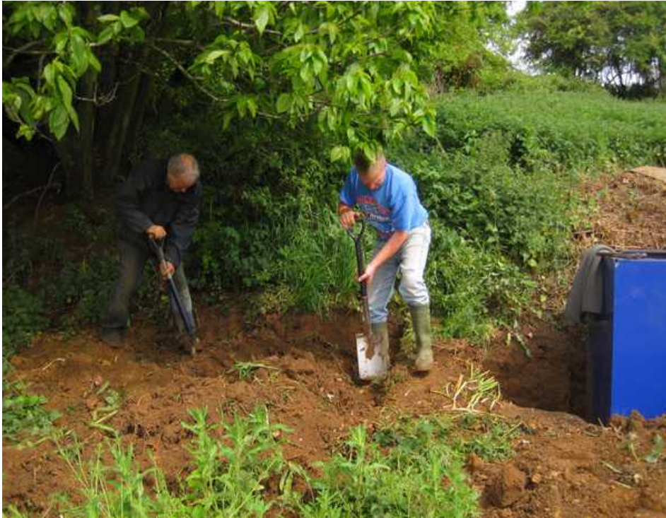
Paul and Nige digging out foundations for the water tanks, now painted & waterproofed inside
