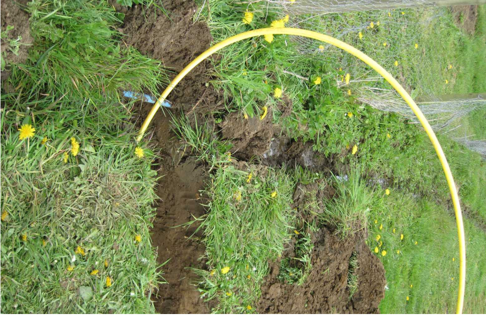
A T-junction in process.
